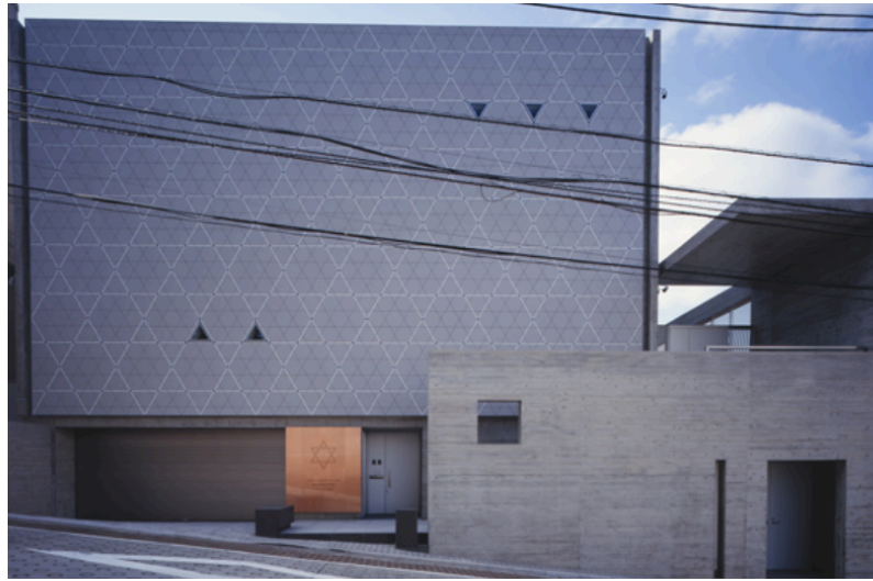
Figure 5. The current JCC building, designed by architect Maki Fumihiko and in use since the early 2000s. Photograph taken in June 2024 (Rachel Fel).
